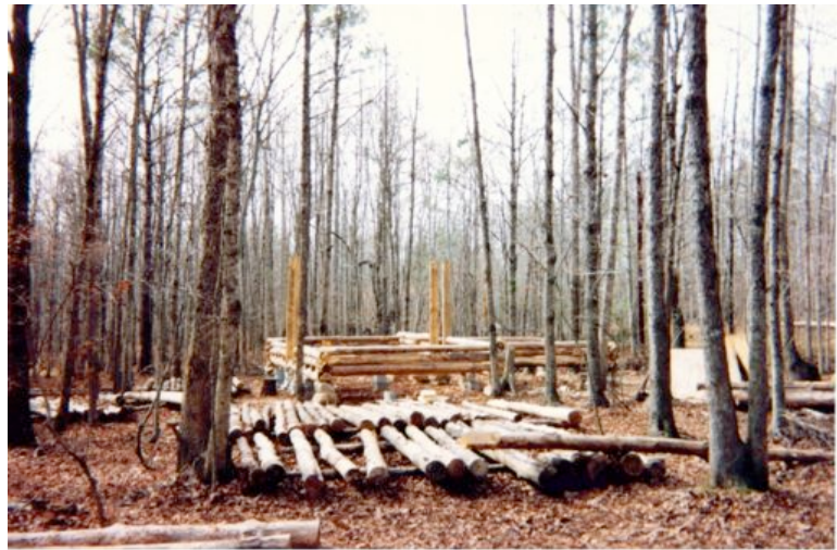
My home under construction, ca. 1991.
